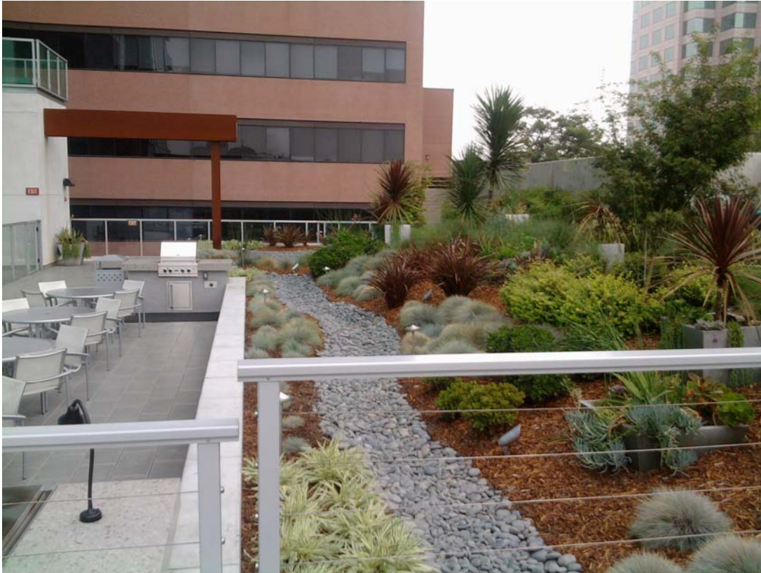
(Watermark Tower—705 West Ninth Street, Los Angeles—2,100 sq. ft. bio-filtration system)
