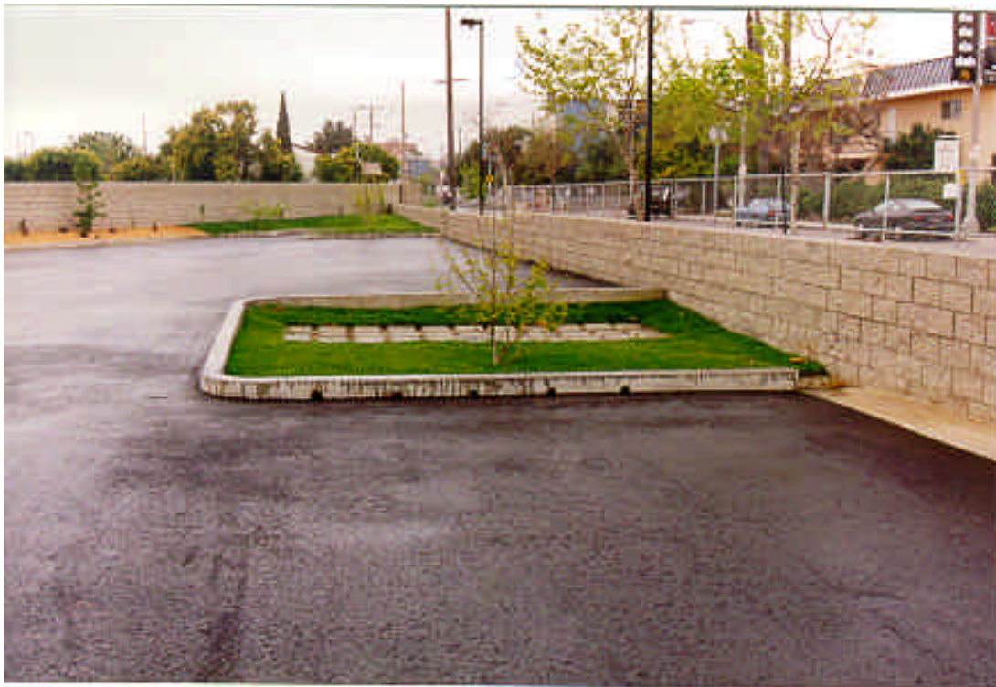
FIGURE 7 Example Infiltration Trench
