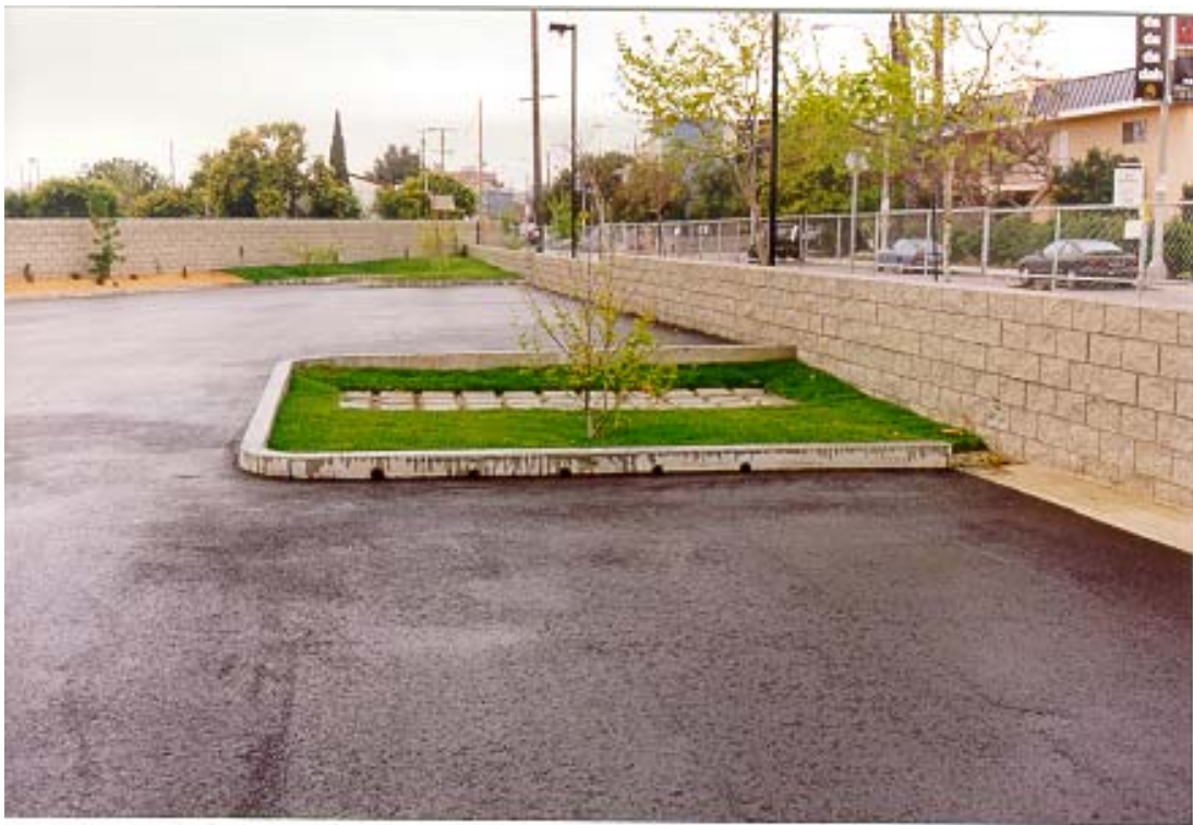
Figure 5 Example Infiltration Trench
